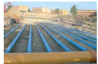
REHAU ground-air heat exchange pipe in grid layout provides sufficient air flow volume for the supermarket's fresh air requirement.
